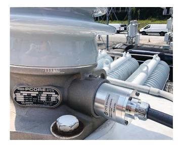
Transformer bushing failures are considered as one of the major causes of transformer outages. Historically, bushings were tested with off-line methods to measure the capacitance and dissipation/power factor.
